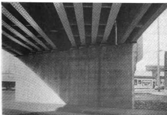
A View Underneath the Brent Street Under-Crossing, Showing the Double-Girder Concrete Fascias that Support the Trainmen's Walks
