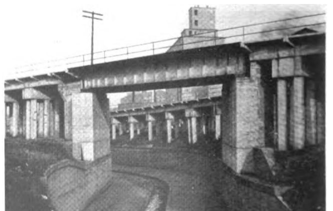
The Beargrass Creek Crossing North of Broadway—Industrial Lead in Background
