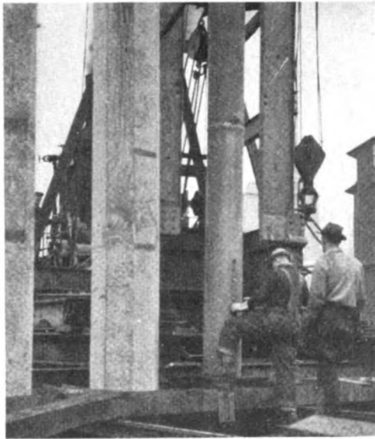
The Pile Driving Outfit. Showing the Pipe Used to Core Holes in Locations Near Existing Substructures
