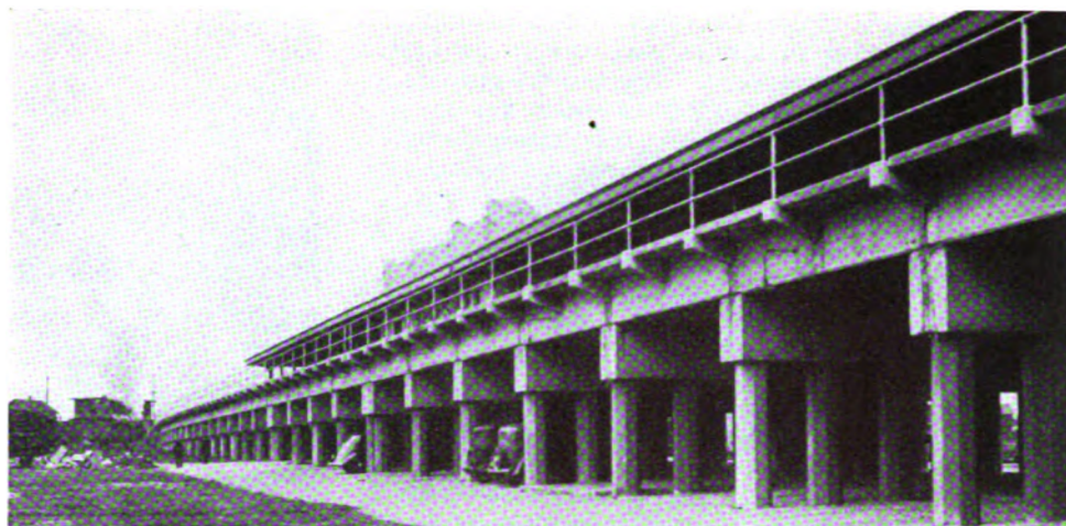
The Concrete Pile Trestle as a Track-Elevation Structure—at the Baxter Avenue Station
