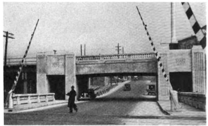
Breckenridge Street Looking Across the Beargrass Creek Bridge Toward the Undercrossing—Automatic Gates for Industry Lead in Foreground
