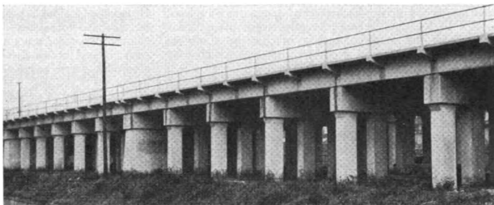
A View of the Trestle Where Cast-in-Place Bents Were Substituted for Pile Bents
