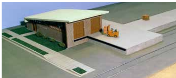
Fig. 16 Street side. A small lawn and some shrubs finish off the street side of the building. The black line along the concrete dock edge is a heavy timber truck bumper.
