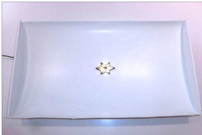
36. Here is the completed 4800-watt star installed in the waiting room roof.
