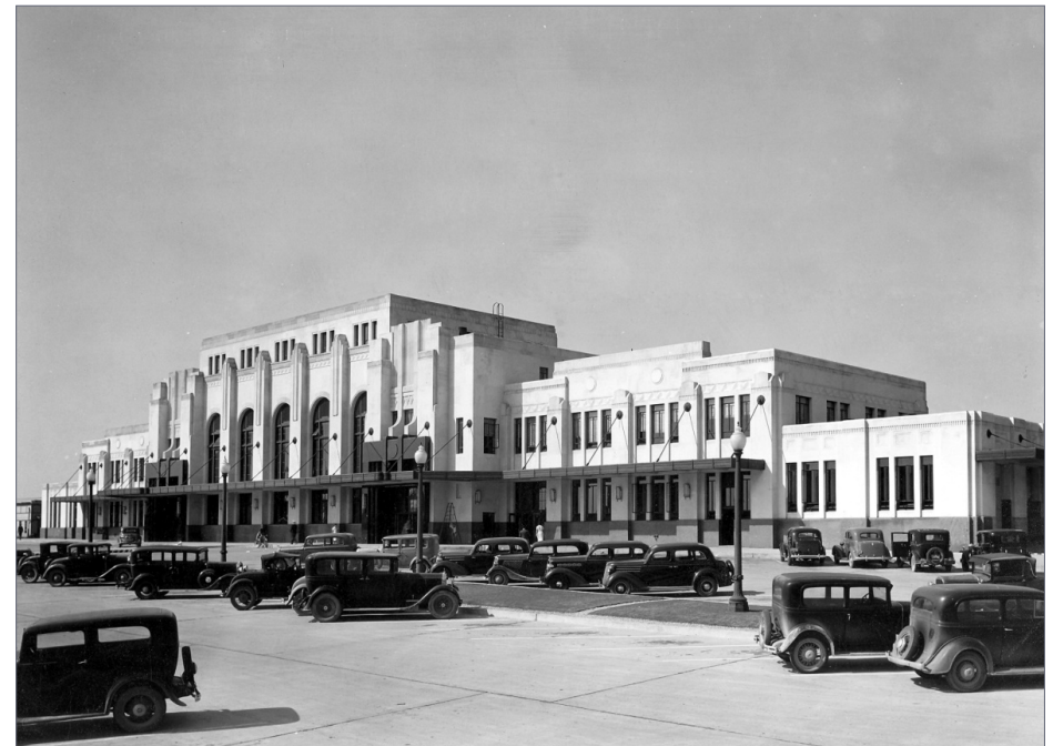
1. Southern Pacific's Houston Grand Central Station shortly after its opening in 1934.
