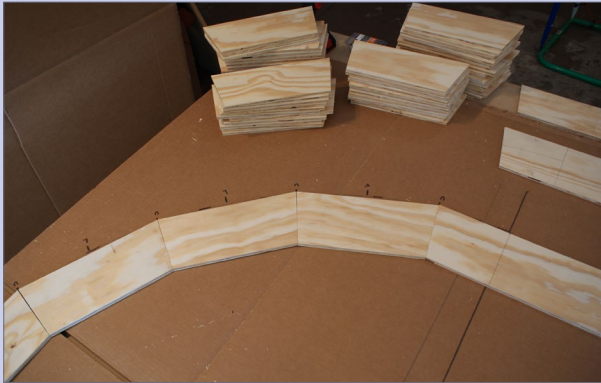
12. Assembly began by aligning the outer edge of the trapezoids on the appropriate marks.
