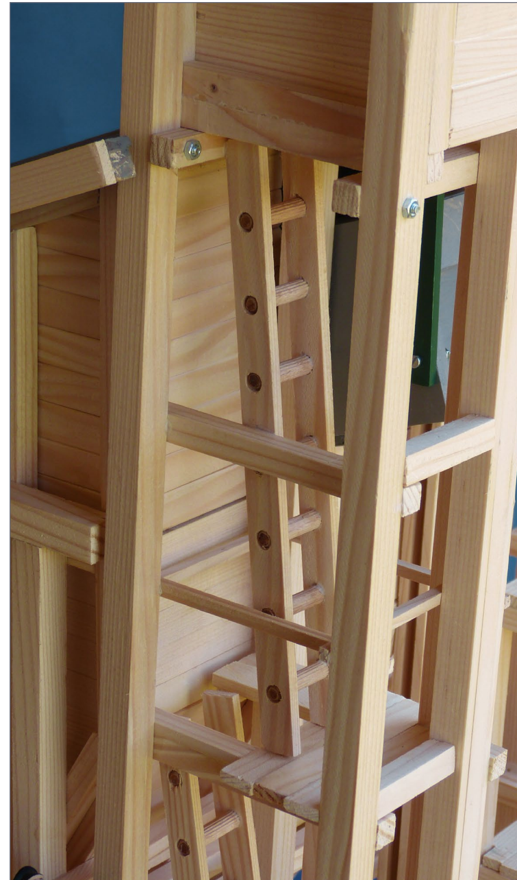
23. Hoist tower assembly, with ladders inside.
