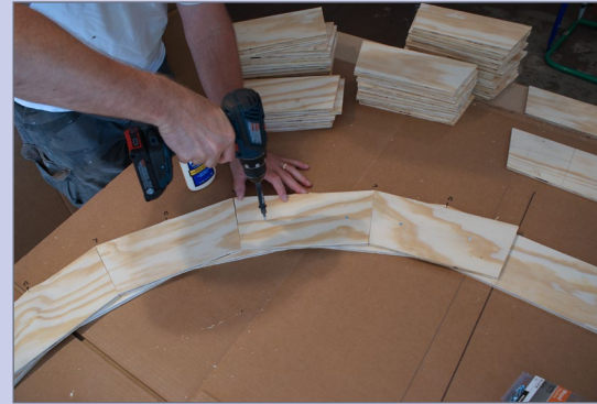
14. I added the upper layer of trapezoids (again using the alignment marks on the outer circle) and used #4 screws to hold the pieces together while the glue cured. In most cases, two screws per trapezoid were sufficient to keep the pieces in place and the joints tight. Although the screws were flush to the surface, I kept them away from the center-line so they wouldn't affect the trackwork later.
