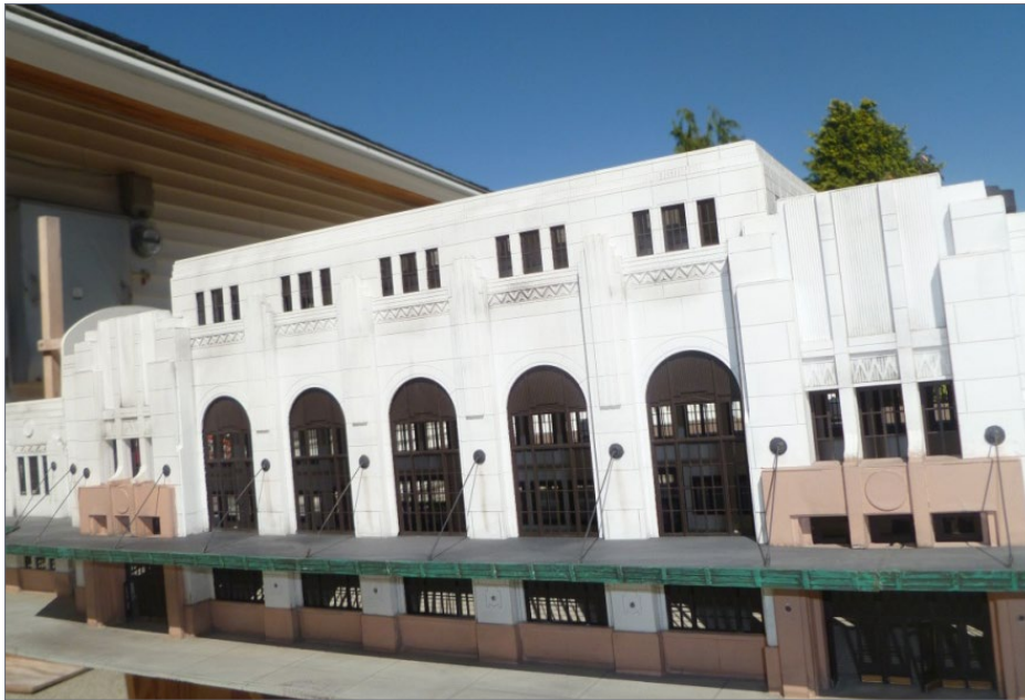
58. The main façade after chalk weathering. It looks convincing.
