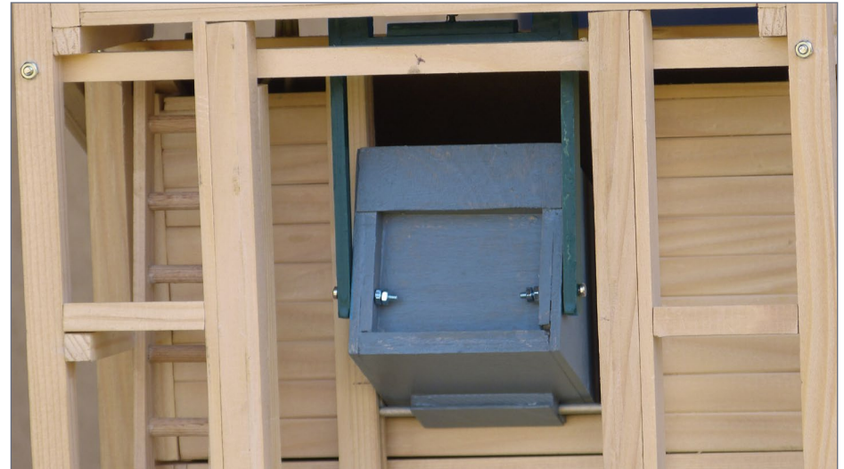
28. Bucket emptying once it reaches the stop at the top of the tower channels.
