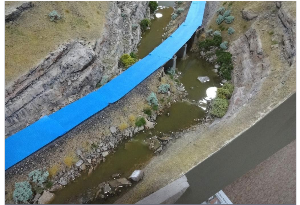
4. Upstream end of the second pour.
