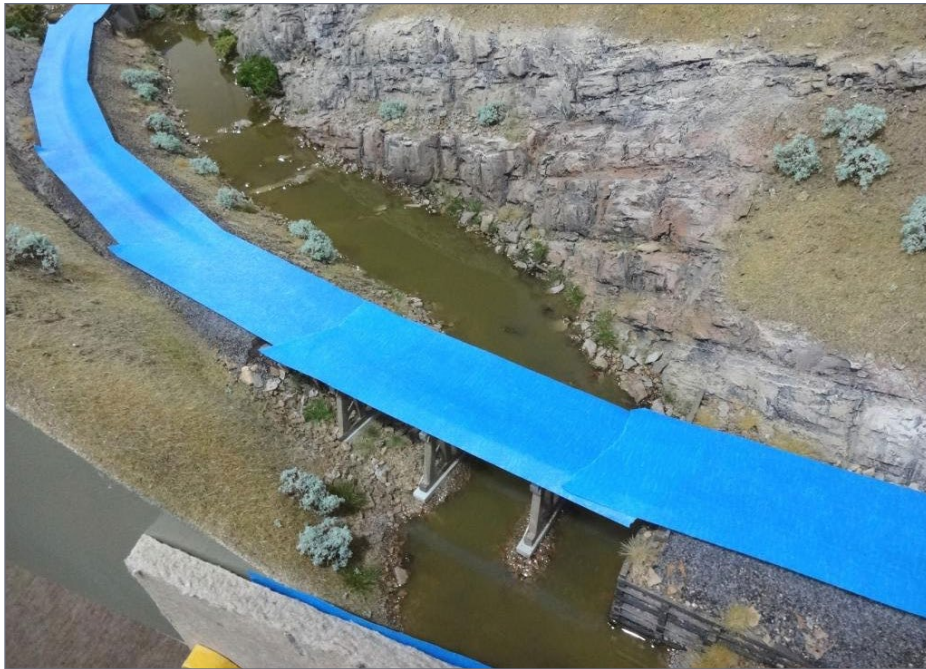
5. Here is the downstream end again.
