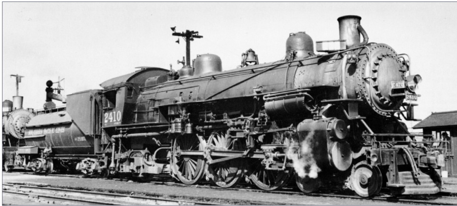
21. This fine portrait of SP 2410, one of the nine locomotives originally classed as P-1 but rebuilt in the 1920s to Class P-4, was taken at the Mission Bay roundhouse in San Francisco in 1946. This engine has received a corrugated-steel pilot, though not all P-4 engines were so equipped. Doug Richter photo
