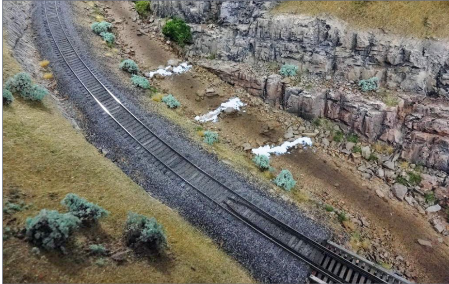
1. Preparing for the first resin pour.
