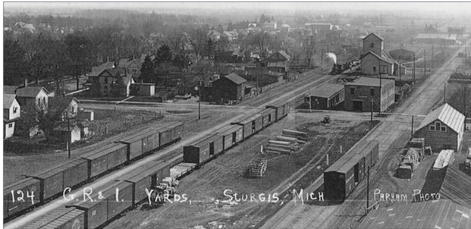
11. Looking southeast at Sturgis, MI over both the GR&I (PRR) on the left and the Michigan Central on the right.
