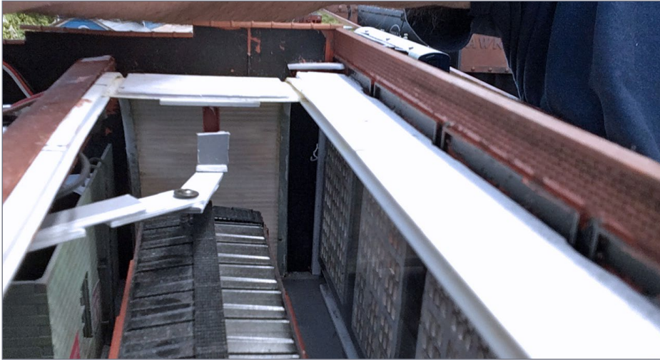
11. The linkage arms and attachment to the underside of the door. You can see some of the patchwork linkage arms where adjustments were made for smooth operation.
