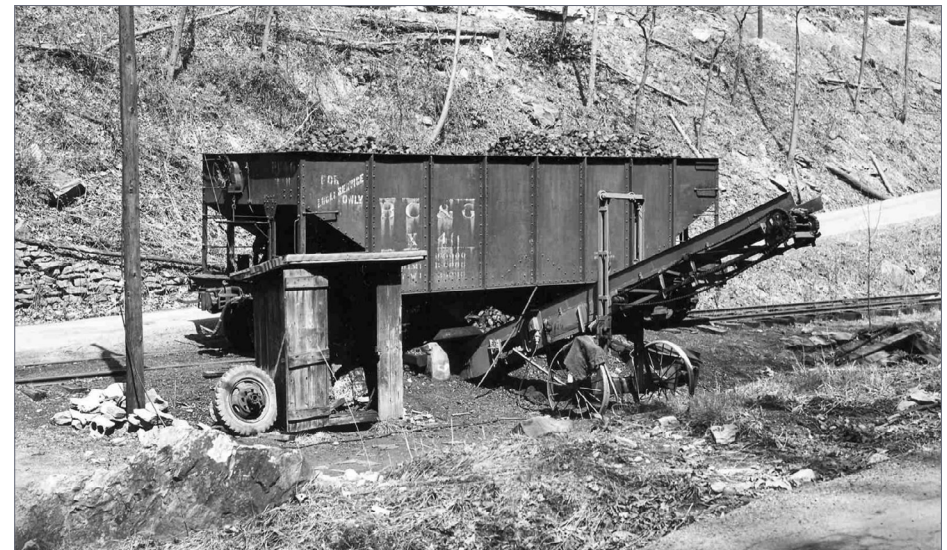
14. Another small coal unloading facility, perfect for a steam-era layout.
