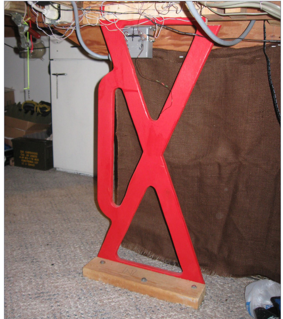
9. We cut out the carpet and mounted this 2x4 directly to the concrete floor on the "Arnold Yard" side. Three lag screws with concrete anchors plus Liquid Nails hold this 2x4 stoutly to the concrete. The red X leg is 7-ply plywood. We similarly anchored a 2x4 and plywood panel on the "Howard" side as well [2].
