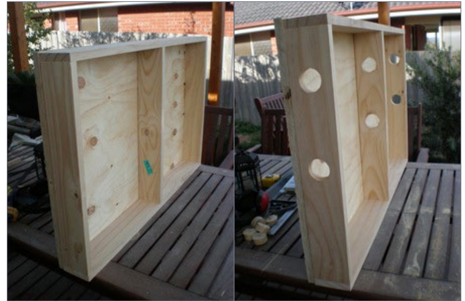
2. The pine frame constructed with plywood top.
