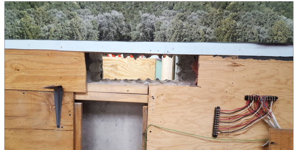
11. Cutting through the plywood at the location in [9] reveals the already drilled holes through the house foundation into the former oil tank room, now Crestwood.
