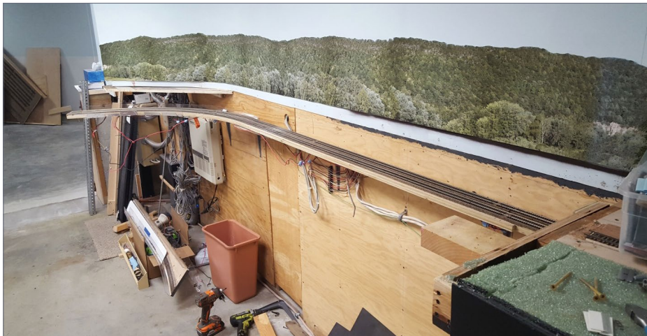
9. This is where Ransom used to be. That staging track curving to the left was later totally removed so the new path to staging could swing out to the right, through the wall.
