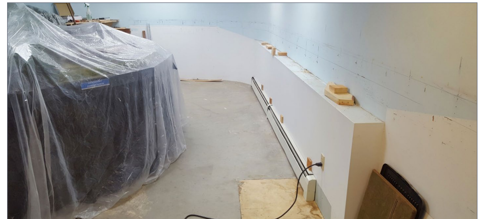
16. This is the old staging and Pittson yard location – and future home of Dupont. Mehoopany is under wraps to the left.
