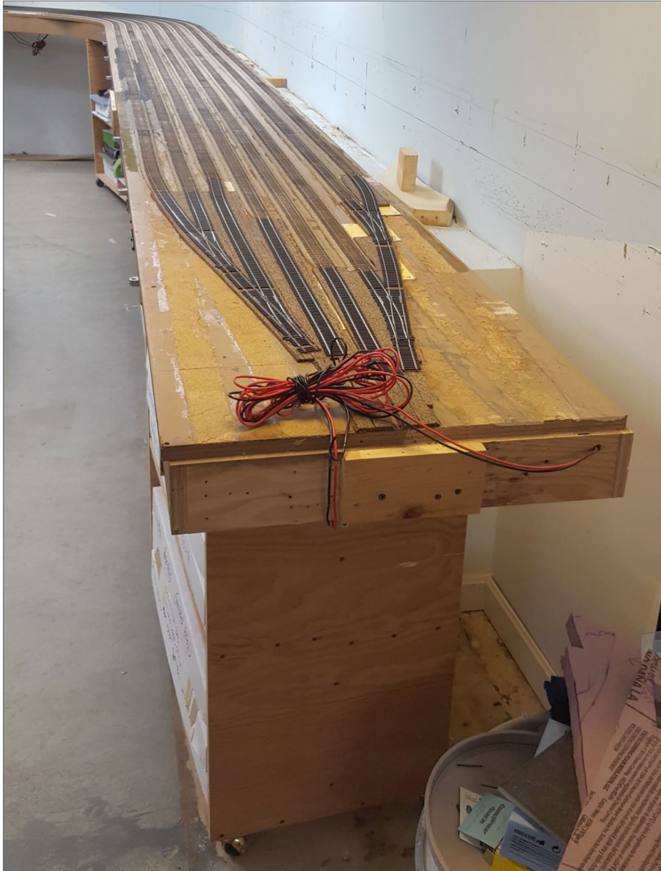
14. The yard is now fully disconnected and supported entirely by the carts and adapters!
