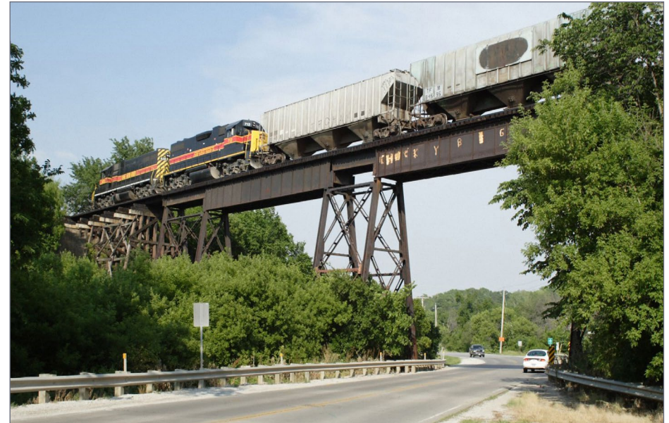
2. In a scene that might be more reminiscent of the Appalachians than Iowa, an eastbound IAIS extra crosses the High Bridge on June 5, 2006. Clean power and picturesque scenes are common hallmarks of the Iowa Interstate. Erik Rasmussen photo
