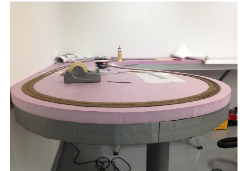
Steel and XPS benchwork.
