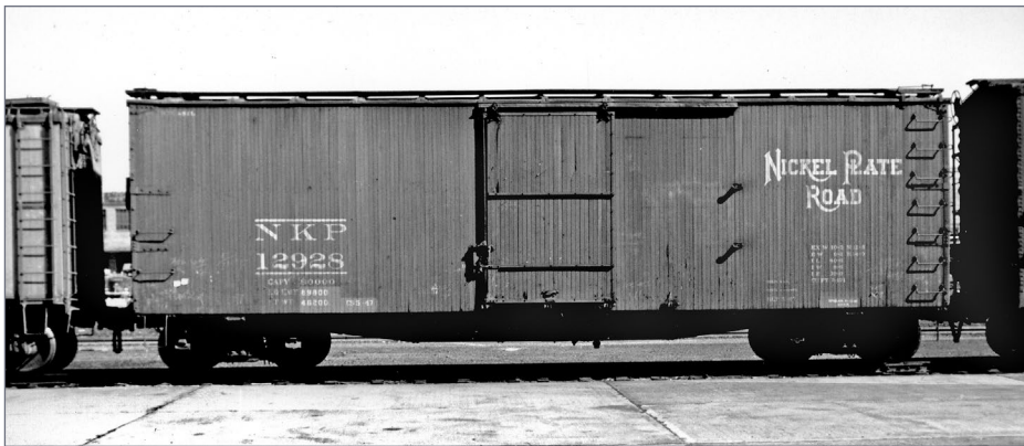
21. Nickel Plate 12928 looks like a USRA double-sheathed boxcar but was built in 1924 as a door-and-a-half automobile boxcar. It's seen here in later years after rebuilding and renumbering. These cars were about a foot taller than the USRA boxcars. Howard Ameling collection, NKPHTS Archives
