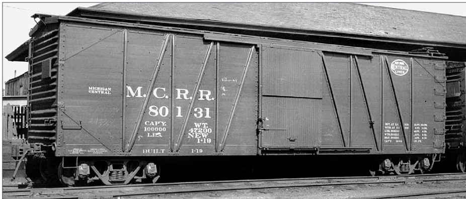
10. This is the inspiration for my Michigan Central (MCRR) model; a USRA single-sheathed boxcar with a straight center sill. This car was built in January of 1919. Ray Breyer collection
