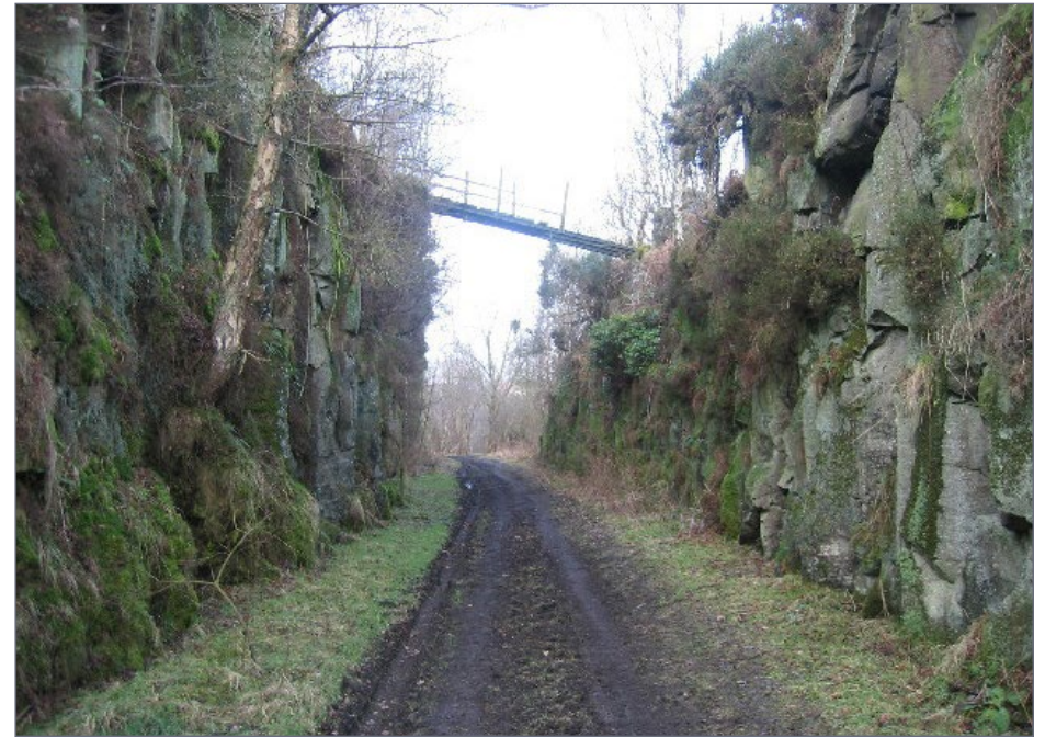
11. This part of the former Rothbury branch is now a hiking trail. A sheep crossing bridge spans the cut. Image from www.geograph.org.uk/photo/124430
