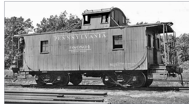
9. PRR 980804 is an N6 with the offset cupola. The lettering follows the practice that started in 1926 or 1927. Note the arch bar trucks with leaf springs. Photo from
