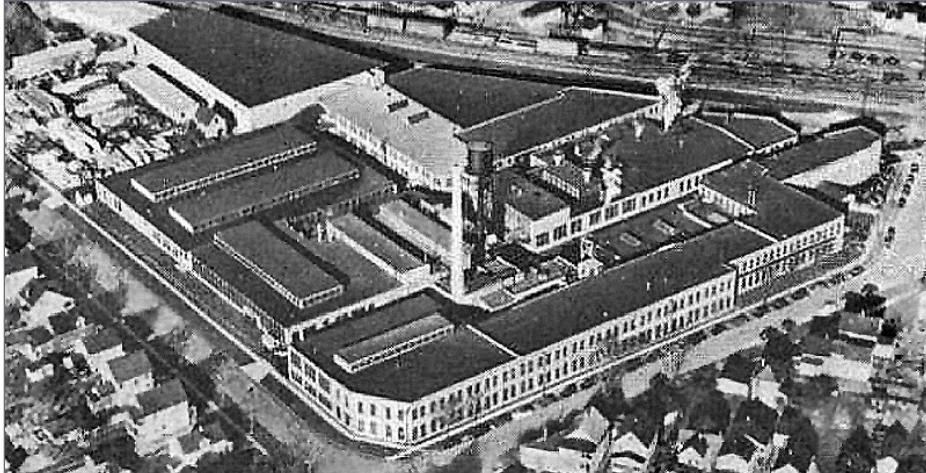
25. It's amazing that this stove works was such a vibrant facility in 1948, the year I was born eight blocks from here. Today there's hardly a trace of this former greatness. American Stove Company 1948 Annual Report
