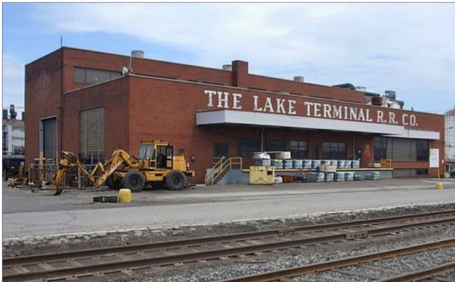
14. Another view of the Lake Terminal offices and diesel house on the National Tube property, not far from the west end of the site. Steve Nathan photo
