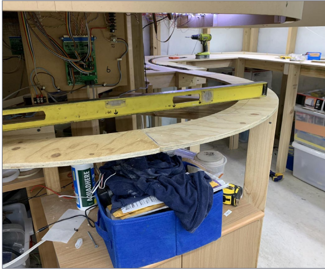
42. Checking the level of the installed loop sections.
