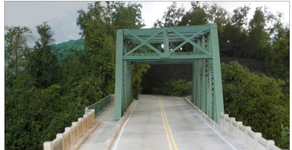
22. Here's your view "driving" down Rt. 11! The culm (waste coal) pile in the right rear is a distinctive element in the prototype scene.
