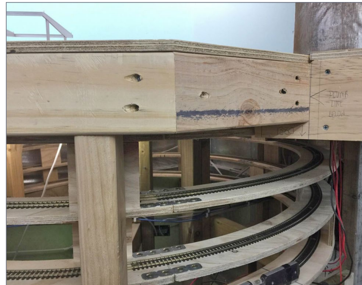
16. The helix underneath the newly installed layout plywood, and the new timber for the fascia.
