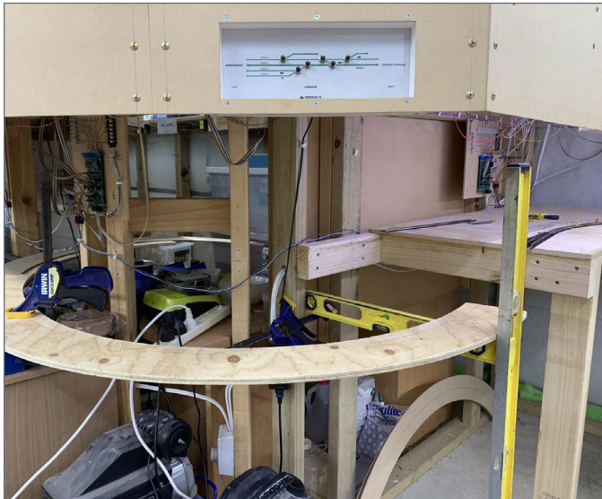
39. Setting up the position of the return loop sections and checking track alignment.
