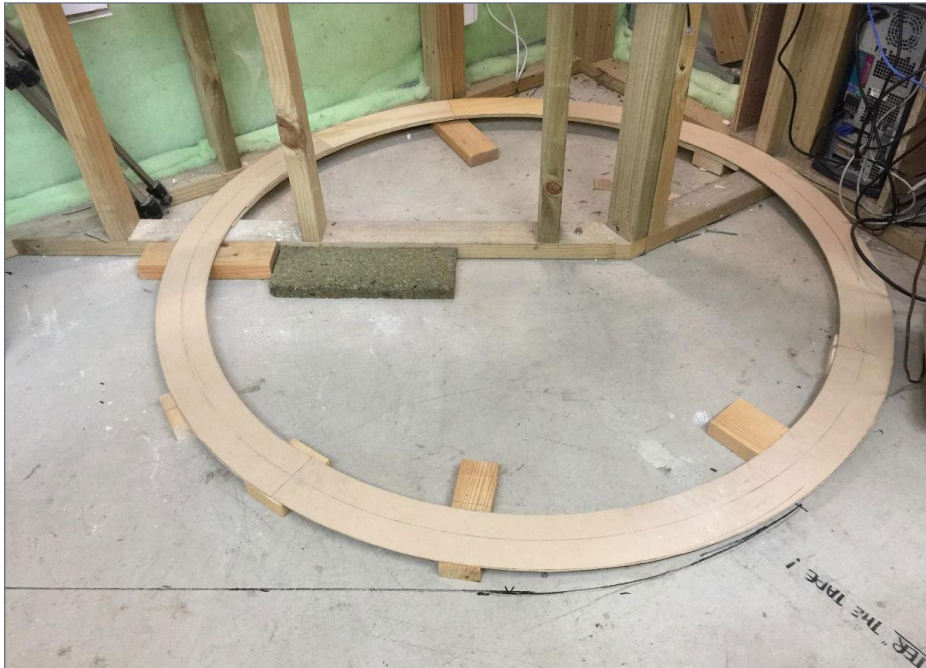
2. MDF templates were used to check the circumference of the helix under the layout.
