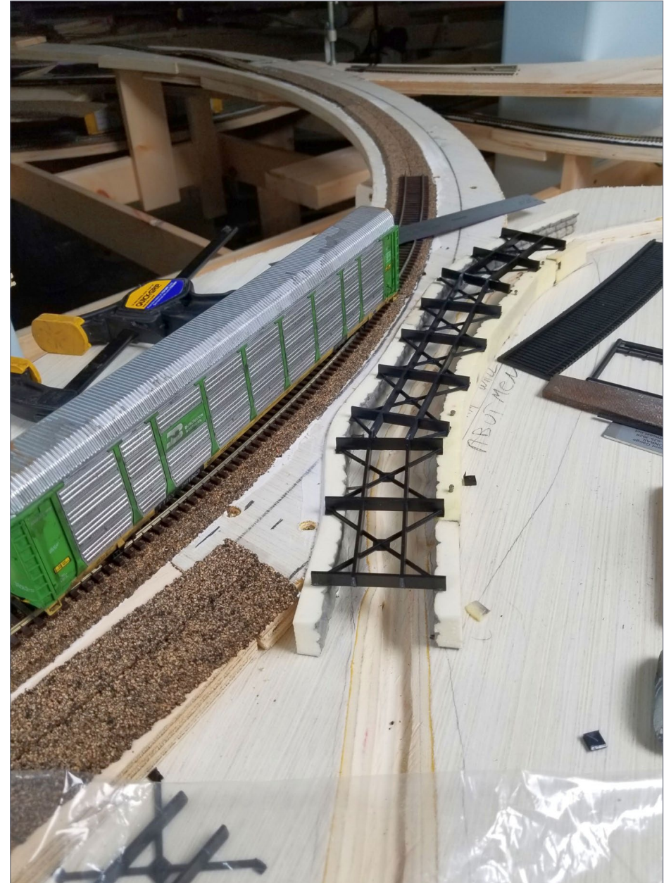
16. Positioning the bridge deck onto the foam walls.
