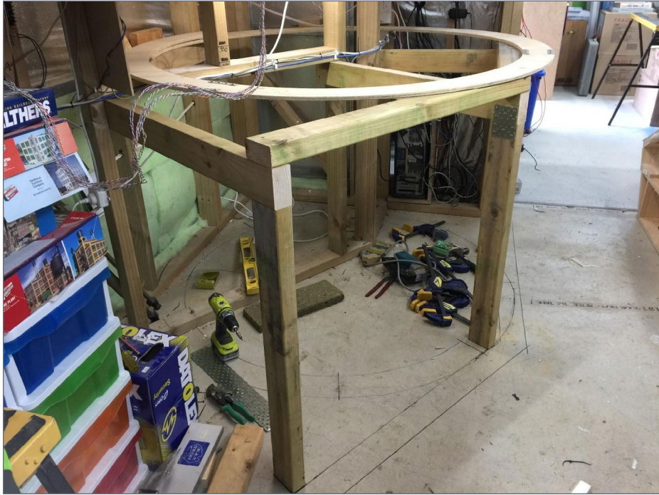
7. The completed helix base frame.
