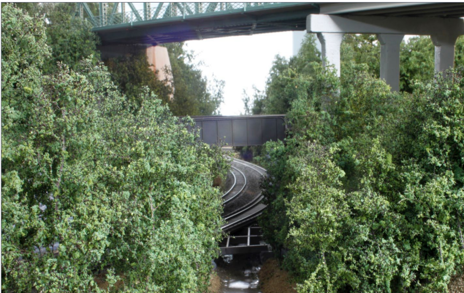
24. This lower angle shot shows the stream going under the tracks – more like what a person would see when standing here.
