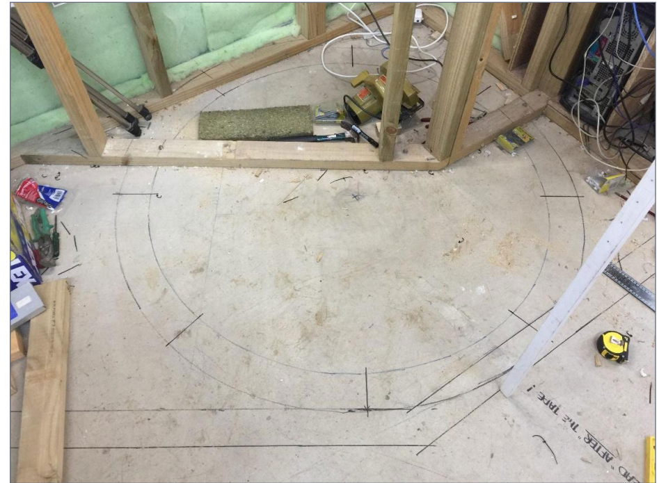
3. The helix position marked onto the concrete floor with the new support structure to be built to support it.
