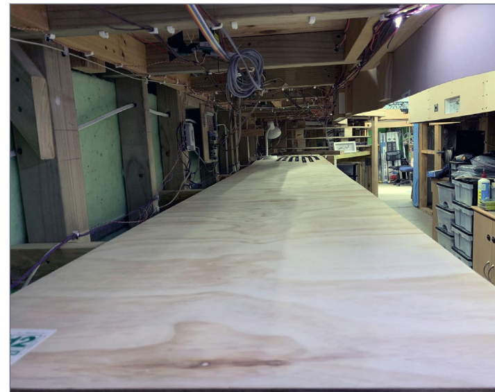
20. The completed north section of the staging deck frame-work and base.
