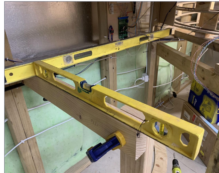
17. Jason's framing timber support legs.
