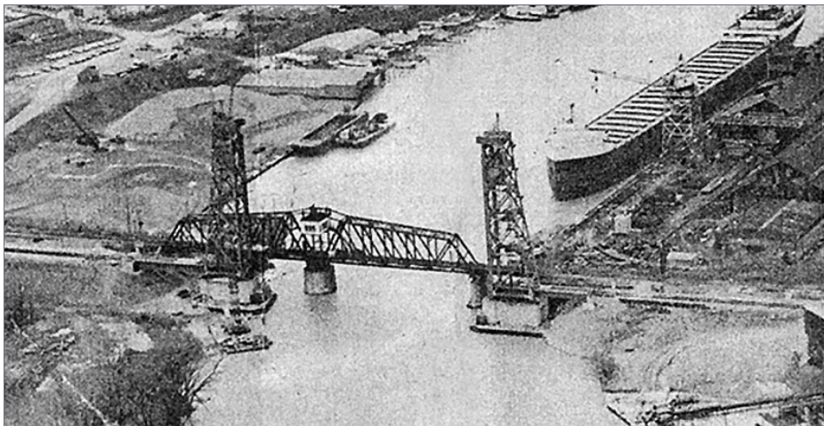
41. The swing bridge lasted until the mid-1970s when it was replaced with a lift bridge that is in service today. The lift bridge progress is documented in this image. Lorain Journal photo
