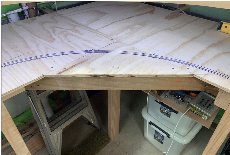
28. Using an alignment gauge to set the radius ensures a perfect curve.
