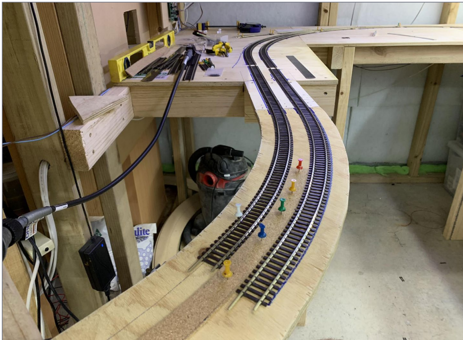
46. Setting the inner loop radius by using the cork spacer.
