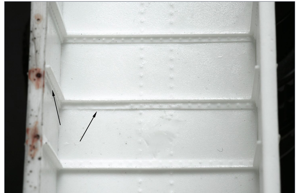
8. Arrows show the rivets removed from the vertical rib and both faces of the floor rib.
