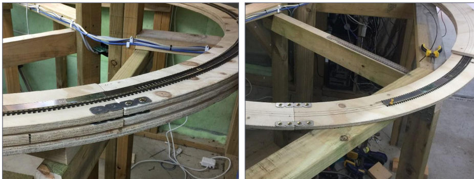
8a & b. The stitching plates and screws used to secure the helix sections.
