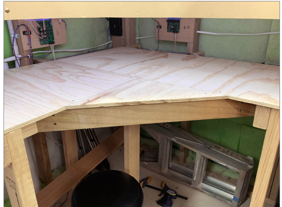
27. The corner section of framework and plywood base.
