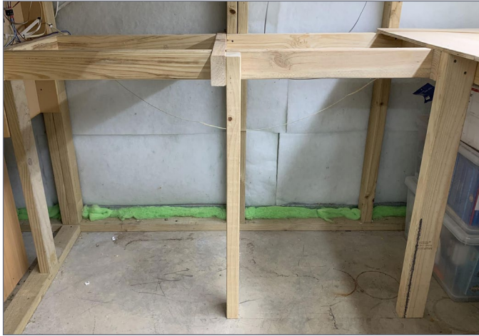
36. The pine framework for the last section bears the 30" radius curve to the return loops.
