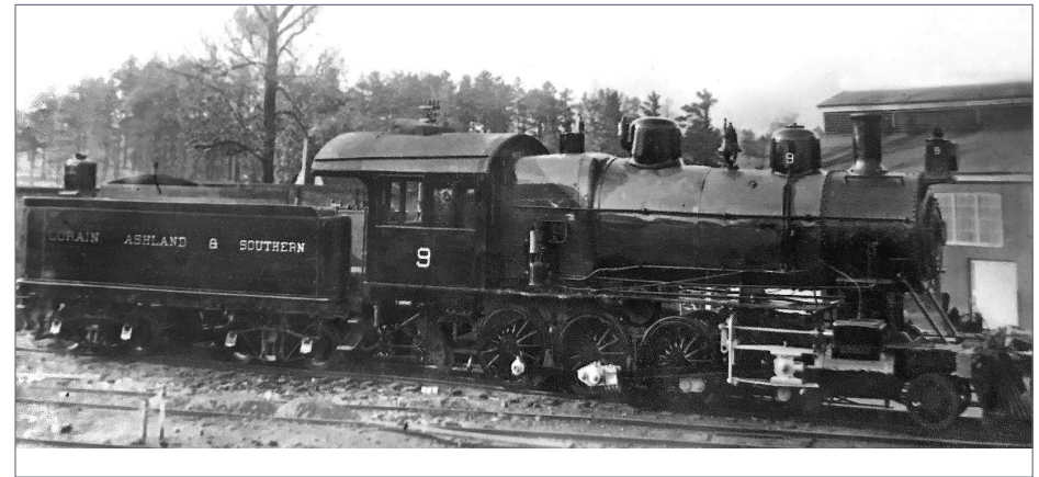
8. LA&S #9, former PRR 6310, H-class hand-me-down. Bridges on the north end of the railroad were too light for larger locomotives. The bridges were not upgraded due to a business downturn in the 1920s. William Snyder, The Rattlesnake and the Ramsey
