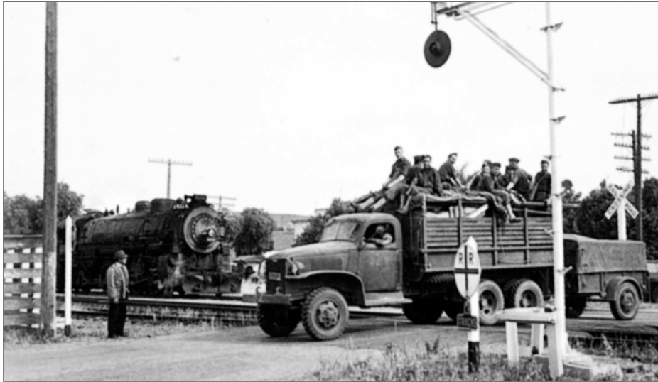
27. This photo was taken during arrival of troops at San Lucas, California in May 1940, en route to Camp Roberts for maneuvers preparing for wartime. The foreground siding track crossing has a wig-wag on the near side and a crossbuck on the far side, at the main line. Note also the Advance Warning Sign, right at the tracks, with an added sign, "3 TRACKS" on the post. Southern Pacific photo, John R. Signor collection
