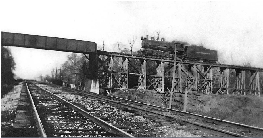
3. This trestle over the B&O mainline near Nova, Ohio, restricted train speeds and weight. One of the leased PRR Consolidations heads north in this late 1916 photo. Note that it is lettered PENNSYLVANIA on the tender. William Snyder, The Rattlesnake and the Ramsey
