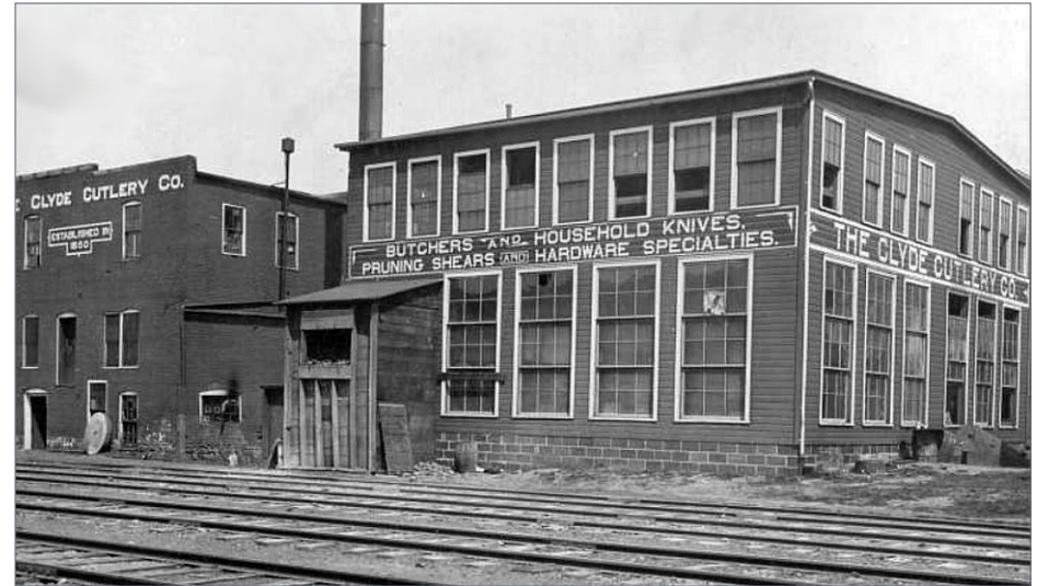
9. Clyde Cutlery was established in 1850. The original brick building is at the left, with a newer, wood building added later. Note the large block foundation and all of those windows. The railroad is five tracks wide in this circa-1890s photo.
