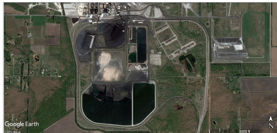
16. The NIPSCO R.M. Schahfer power station in Wheatfield, Indiana, is a massive facility with five full unit train arrival tracks and two full unit train departure tracks. It lies at the end of the NS Kankakee branch line. The facility is slated to be decommissioned in 2023. Google Maps
