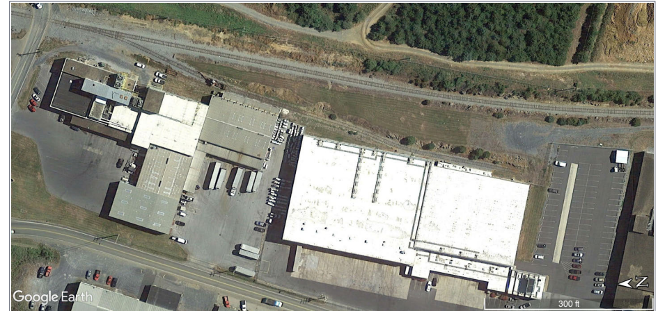
32. US Cold Storage facility in Harrisonburg. Google Maps
