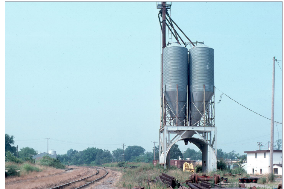
1. Powell Feed and Milling Silo Complex from the north.
