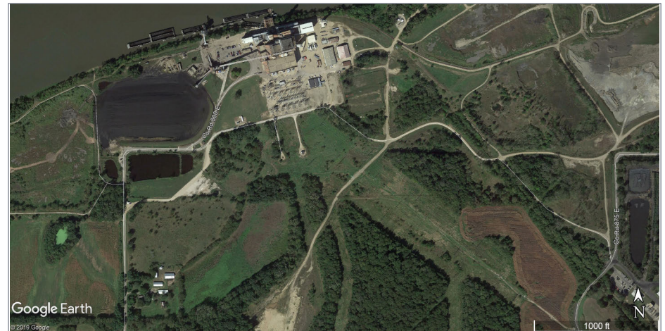
14. Hennepin Power & Energy is a coal-fired power station near the end of the Kankakee branch line. The end of the branch line can be seen just to the left of the compass "N" in the lower right corner of the image. Google Maps
