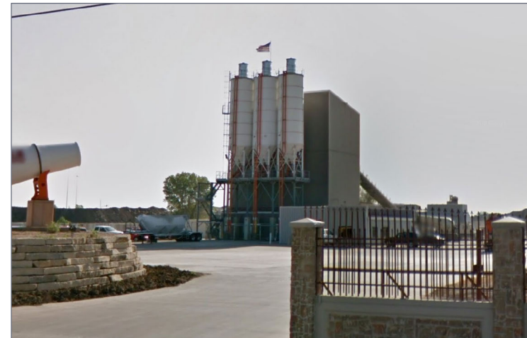
19. Andale Ready-Mix cement silos.
