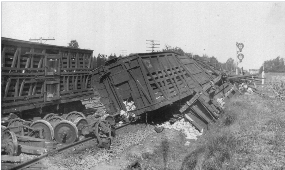
29. This wreck image shows several crushed Lehigh Valley stock cars that had been loaded with cabbages.
