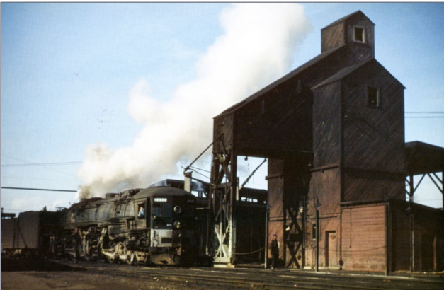
10. Some sand houses were truly large, such as this one at West Oakland. It was a major landmark in that yard. But notice the small diameter and unimposing supports for the sand delivery pipe. Barry Anderson photo
