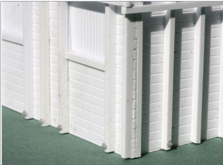
20. Rear corner of sand house, showing appearance of boards sandwiched between posts at corner (compare [12], and NBW in place.
