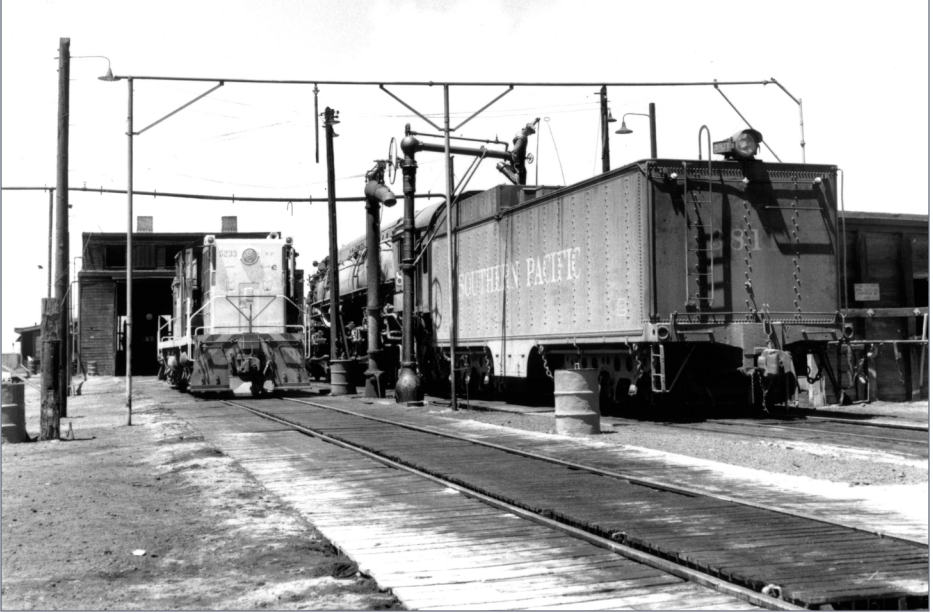
5. The sand house at Wendel, California, just visible to the right in this 1951 photo of the engine terminal, also had no tower. That rickety-looking piping over the track is for sand delivery. Richard Steinheimer photo, DeGolyer Library collection
