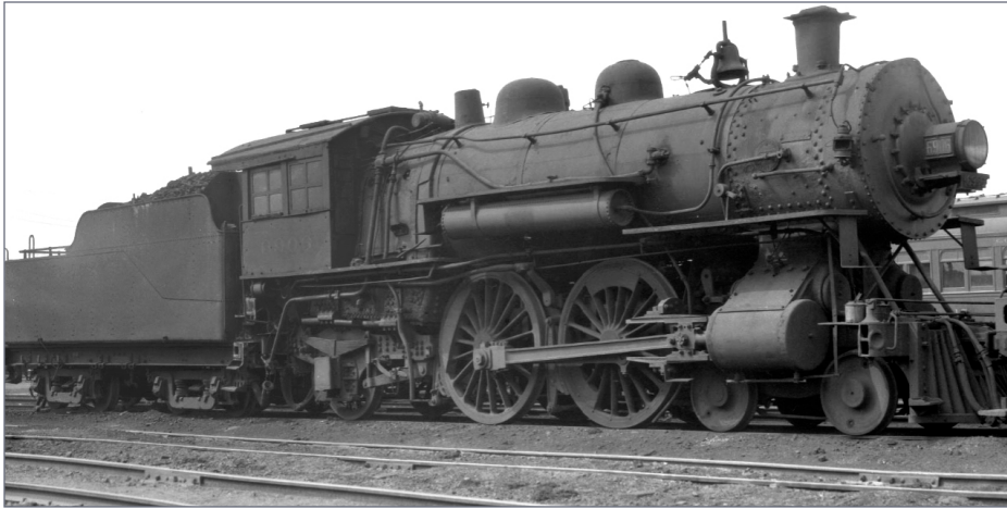
5. NYC 6906 at Indianapolis, Indiana in September 1927. This I-class Atlantic has an early cab and early slanted cylinders, both typical of a 1900-1910 build. The increased firebox size and larger boiler made the Atlantic a significant improvement over the earlier 4-4-0 American type locomotives. In the end, they were a stepping stone to the even larger 4-6-2 Pacific. Ray Breyer Collection
