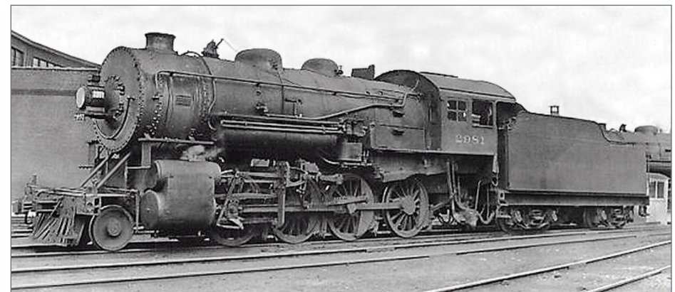
15. NYC Lines 2981 was not a pretty sight, but it definitely was functional. Alco's Brooks Works built this G6 class Consolidation in 1910. Although 2981 was retired and torched in 1932, many of the class lasted into the early 1950s. Ray Breyer collection
