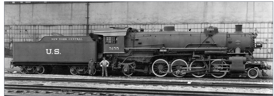
22. This photo of NYC 5155 is one of my favorite steam locomotive photos. It was taken shortly after emerging from the shop and may even be a builder's photo. The USRA Mikado is one of the finest-looking steam locomotives ever produced. It was also one of the most successful, lasting from 1918 to the mid-1950s.
