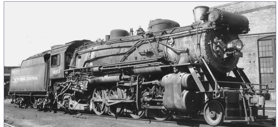
26. It is believed that this is the only NYC USRA Mike fitted with an Elesco feedwater heater. While the test was successful, the railroad abandoned the project due to loss of traffic during the Great Depression. This locomotive looks awesome and I wish more units were converted. This locomotive was originally numbered as the 5153 but was renumbered to 1853 in August of 1935 when the NYC Lines became the NYC System.
