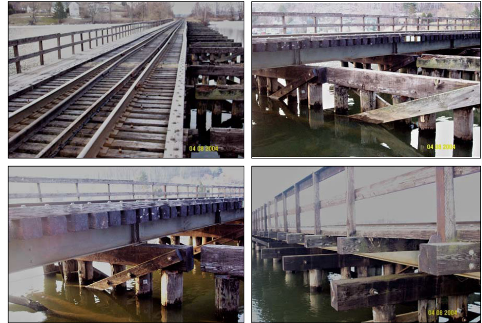
2. (Clockwise from top right) View from the deck reveals that this line was once double-track; now unburdened bridge piers stand in the lake; detailing of the deck's railing and stanchions; closeup of the trestle structure supporting the active line reveals the bolts of the angle bracing.
