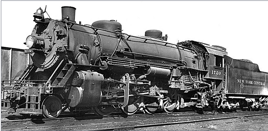
23. The 1720 is almost unchanged since being delivered to the railroad about 1920. These locomotives were so well-designed, reliable, and modern that there was no real need for upgrade. The wind deflectors atop the cab roof were a later addition for creature comfort. Note the poling pole and rerailed frogs stowed underneath the tender frame. Ray Breyer collection
