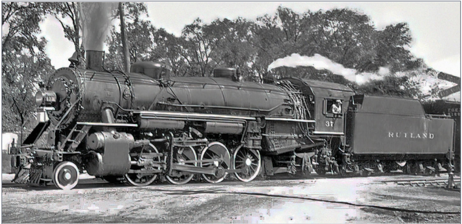
42. Rutland 37 looks like any other railroad's USRA light Mike. All were built to the same USRA design and specifications. After the USRA lost control, individual railroads began to make changes to suit themselves. Ray Breyer collection
