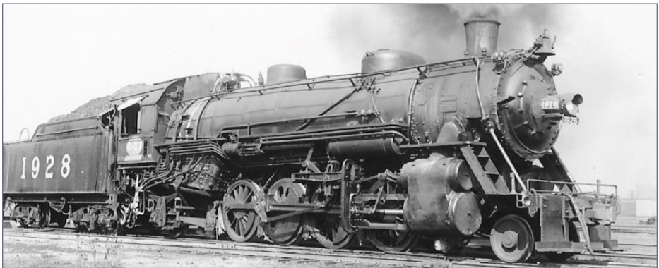
9. C&EI 1928 in a 1942 photo, built by Alco in 1918. She is painted in the later paint scheme. Note the shroud covering some of the plumbing appliances ahead of the cab atop the firebox. Ray Breyer collection
