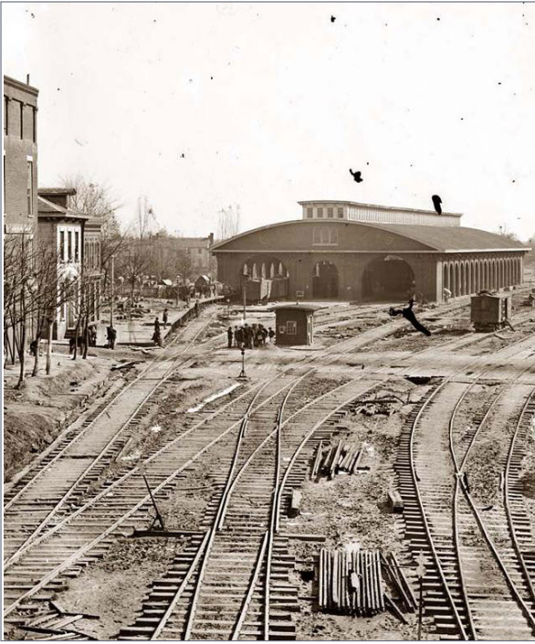
2. Atlanta station approach showing the 5-foot gauge track. Note the two stub switches in the foreground, arranged toe to toe to create a double slip.
