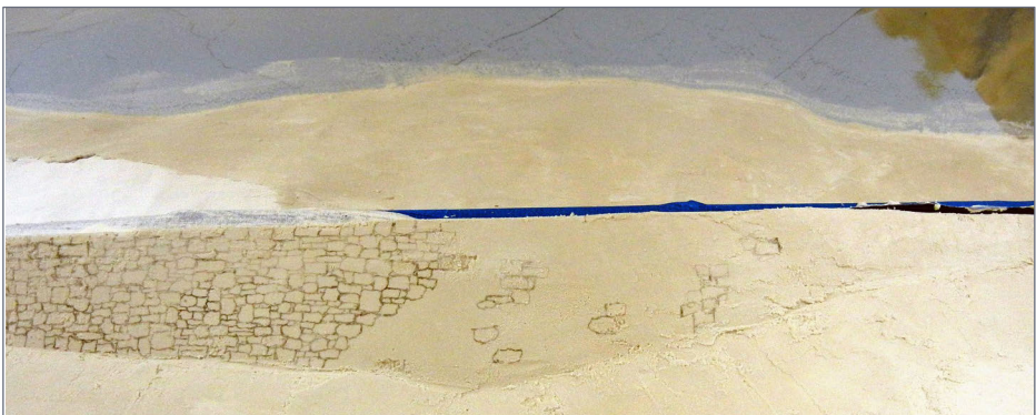
30. Penciling-in the stones on the plaster retaining wall.
