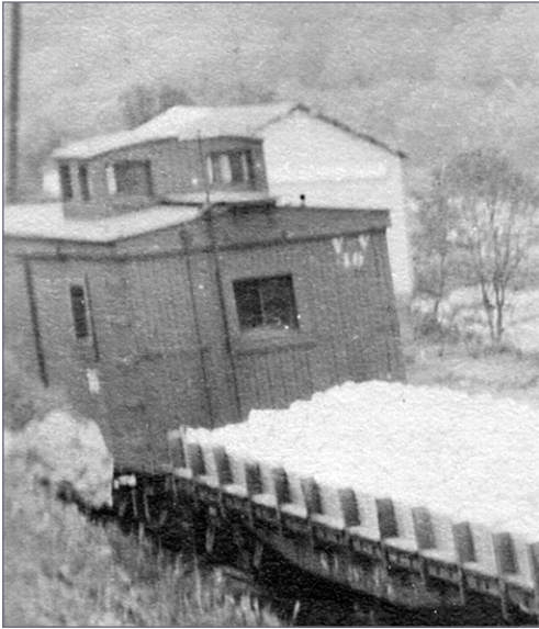
5. The cupola does not extend the width of the roof.
