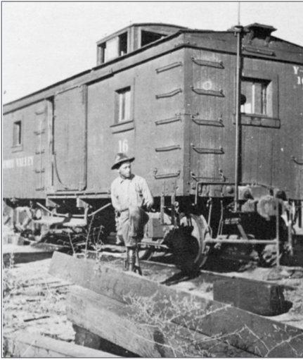
10. This photo of the second caboose No. 16 shows some of the details of the outside-hung brake shoes.
