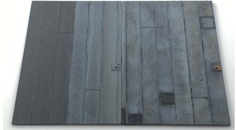
2. Left-to-right: Flat roof nearly new, medium-aged, needing replacement. Note the patched areas where the aging roof has been repaired.
