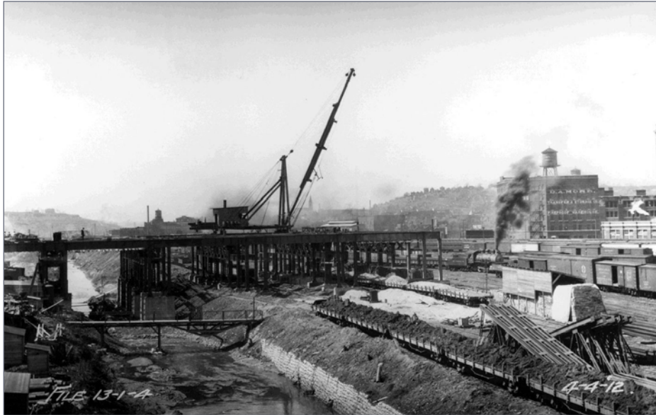
12. Placing support columns for the waiting room.
