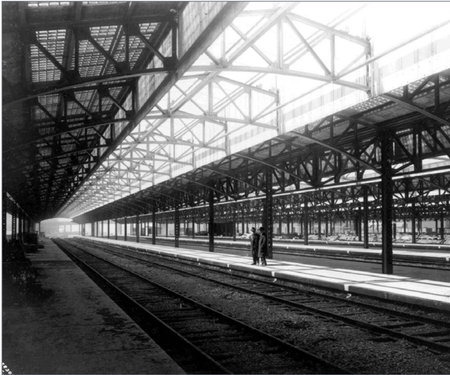
34. The Union Station platform canopies as built. Note the glass block sections.
