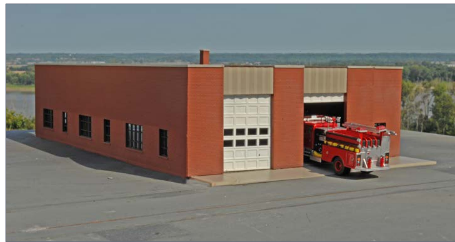
16. The Fire Department Repair Shop building can be used as an industry or utility repair shop or other building that needs to have vehicular access.
