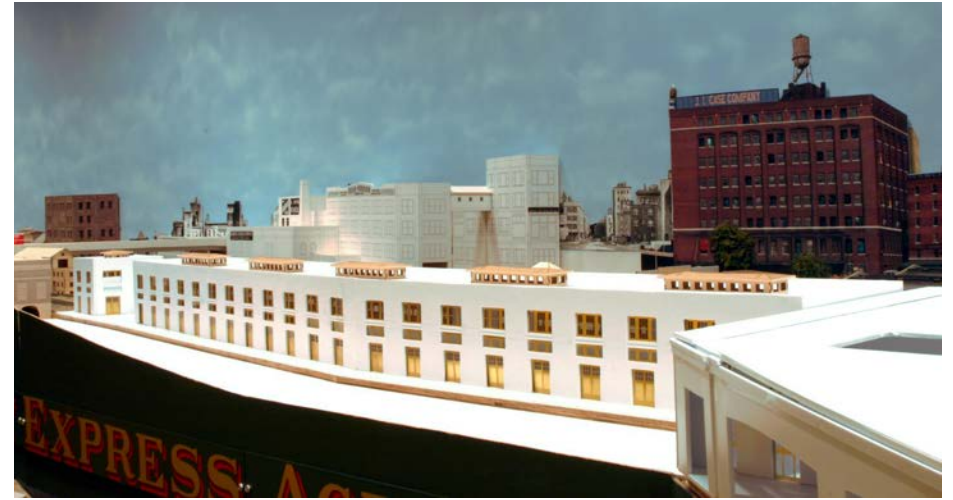
44. The Railway Express building takes shape.
