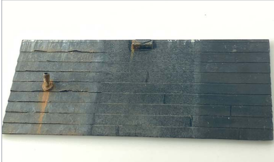
1. Left-to-right: Sloped roof needing replacement, mid-life, and nearly new.
