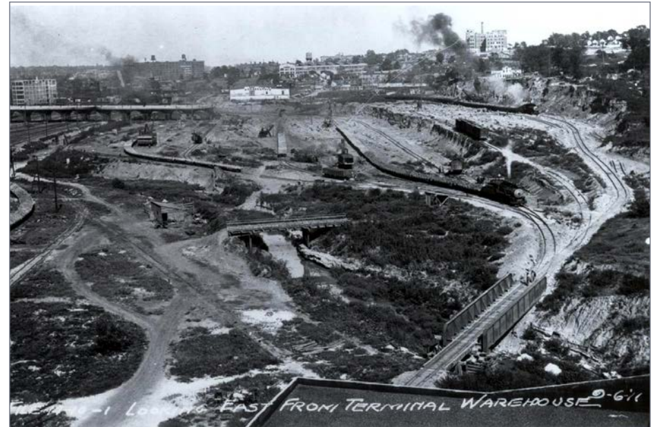
11. Early site preparation. OK Creek can be seen meandering from upper-left to lower-right.
