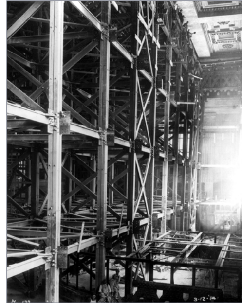
14. Scaffolding ready to be removed from inside the completed Grand Lobby.
