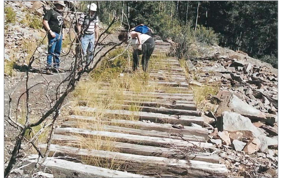
5. 60 years after the rails were pulled, the old roadbed is starting to wash out, but the ties remain. The Forest Service maintains the path at left.
