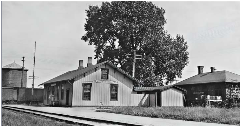
8. Here is the Monroeville LS&MS passenger depot about 1900 looking southeast. A B&O train is crossing the LS&MS. The LS&MS water tower is in the background. Look at the milk cans on the carts in this photo. Trains will have to stop to pick up milk and drop off empties. It's amazing just how much work the railroads did a hundred years ago.
