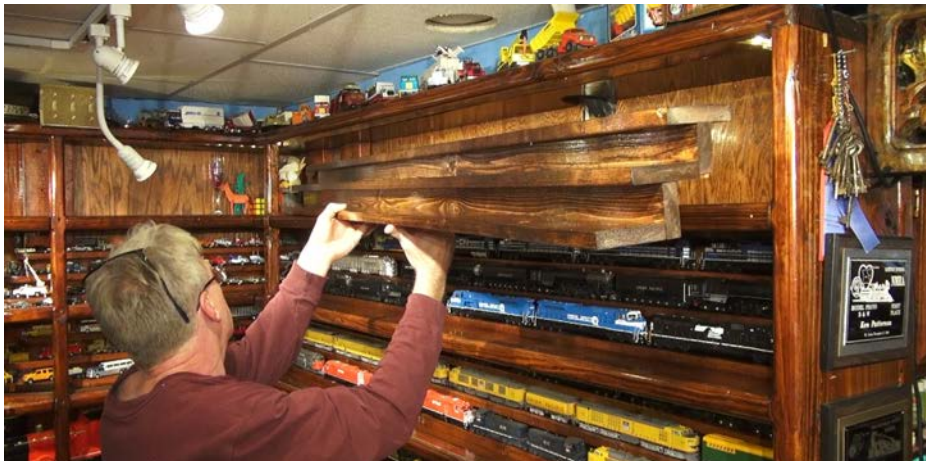
12. The shelf inserts slip inside the openings in Ken's shelves, which were built out of 2x12 dimensional lumber. The shelves are generally screwed down to secure them.
