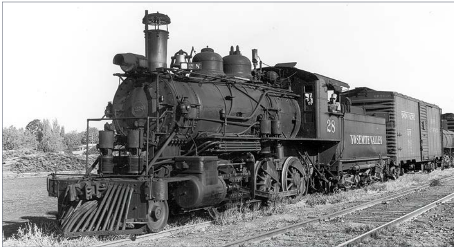
18. The No. 28 in 1942 with the extra pair of air pumps on the front pilot. During the war with Japan in 1941, all of the YV locomotives were fitted with blackout visors over the front headlights. Bob Lunoe photo
