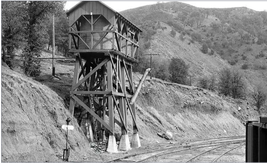
30. This is the last pair of water tanks installed in Bagby in 1939. Todd Pederson Collection
