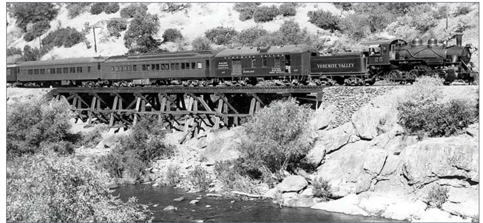
33. This photo from July 7, 1940, shows Train No. 2 crossing Bridge 64A. The train that day consisted of locomotive No. 25, YV RPO car 107, leased Southern Pacific Railroad diner 10300, a Pullman picked up that morning from the Southern Pacific Railroad in Merced, and YV observation No. 330. The observation car still exists today in beautifully restored, original condition. Wilbur C. Whittaker photo
