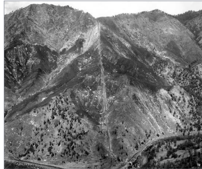
3. The northside logging incline was 8,600 feet long with grades as steep as 6.6% and a 3,000-foot elevation drop. The community of Incline was at the bottom of the incline.
