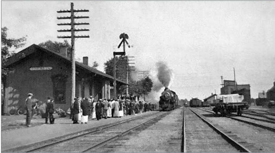
32. Passengers wait on the platform as the train approaches the Oberlin depot from the west sometime circa 1910. Rail-served businesses are at the right. The freight house is in the distance.
