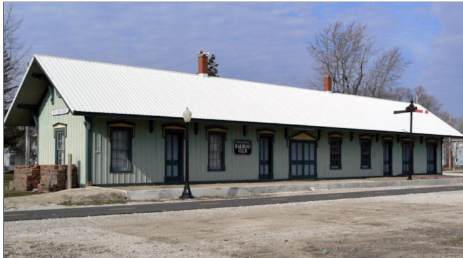
7. Here is the Elmore depot in 2009, restored and serving as home to the local railroad club. It is classic Lake Shore & Michigan Southern architecture. Compare with the Genoa depot in [6].
