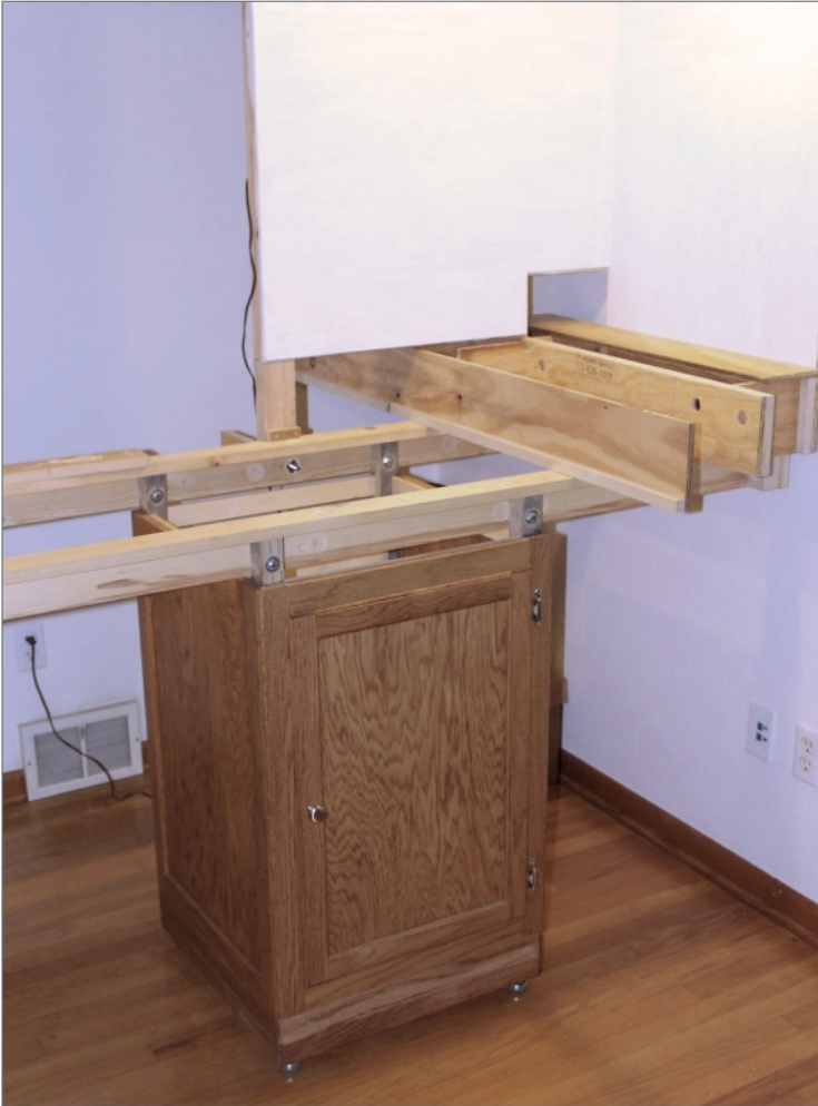
9. Typical placement of a benchwork-box under a section of a layout.
