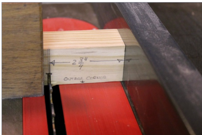
6. First saw cuts across the leg to form one side of the slot.
