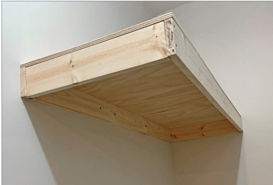
8. The first layout section attached to the walls, but not yet supported from below. That is next. On later sections, I installed the knee brace before the plywood deck.
