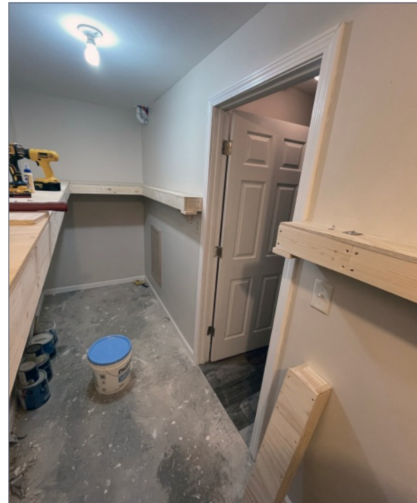
20. The bridge is leaning against the wall. I plan to install a wall bracket to store it when it is not in use.
