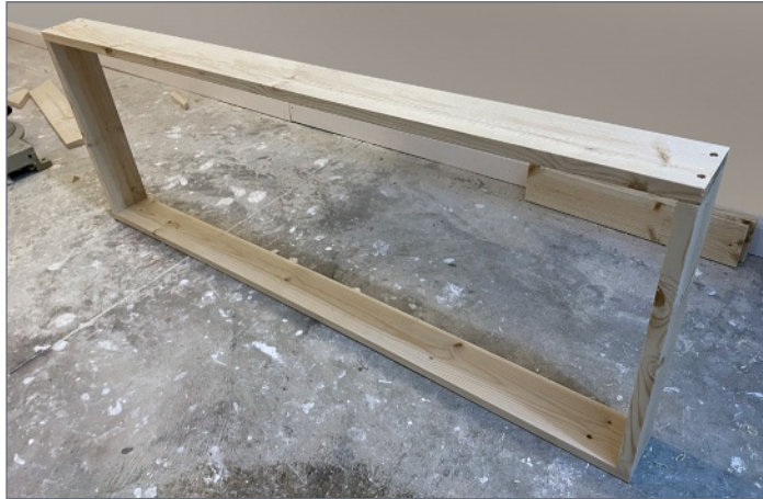
7. The frame of the first 4'x18" layout section. The ½-inch thick poplar plywood top made it more than strong enough without additional bracing.
