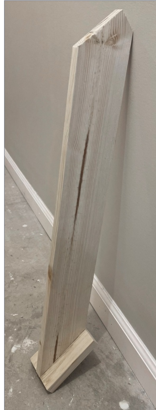
9. One of the knee braces that will be installed to support the layout shelves [10, 13]. I used my chop saw to cut the 1x4 lumber for these knee braces.
