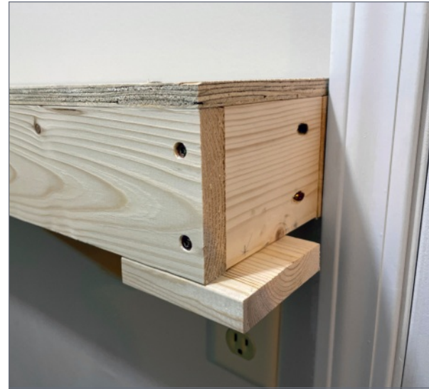
19. I built bridge supports on either side of the door. I will round the corner so it does not have a sharp point that might hurt someone. Screws hold all wood sections together.
