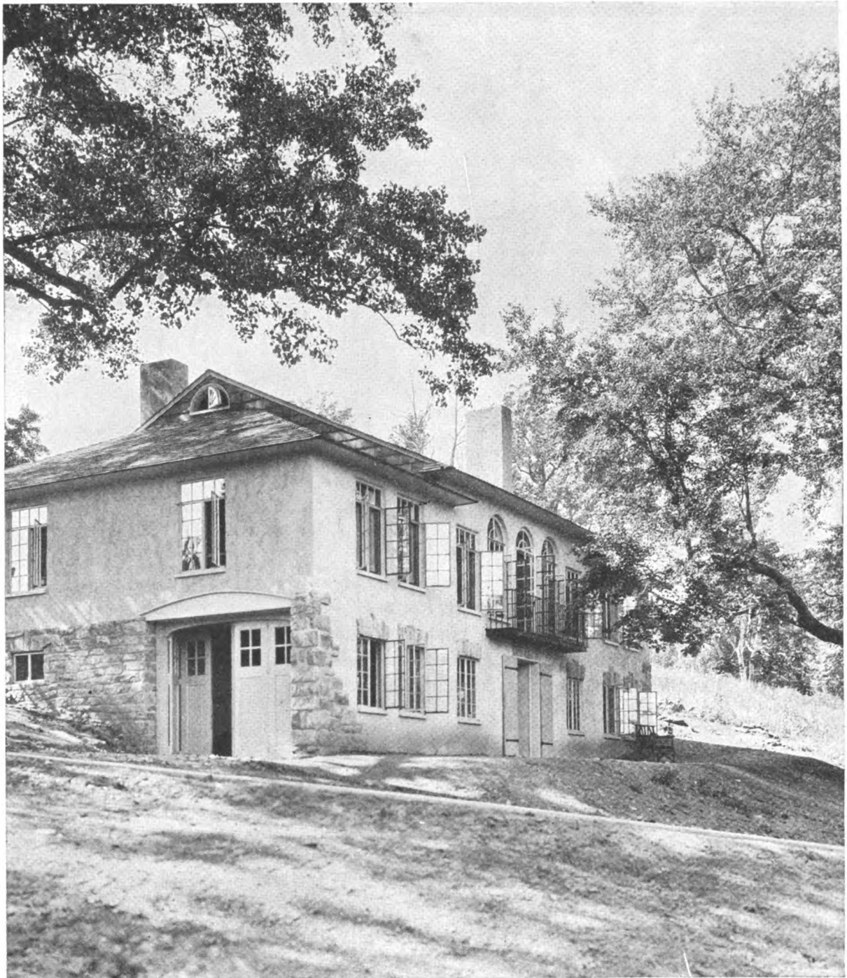
The Charles W. Garrett Residence Wallingford, Pa.
