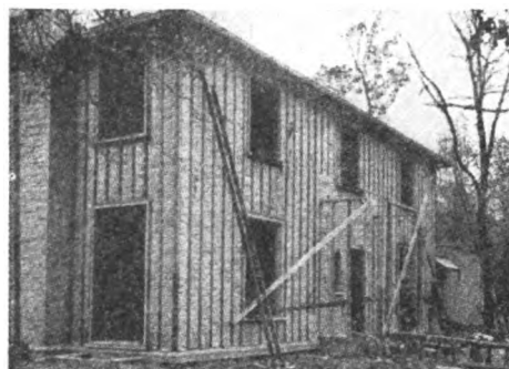
This shows a house insulated with Cabot's Quilt, ready to receive the outside finish. Russell S. Walcott, Architect, Chicago, Ill.
